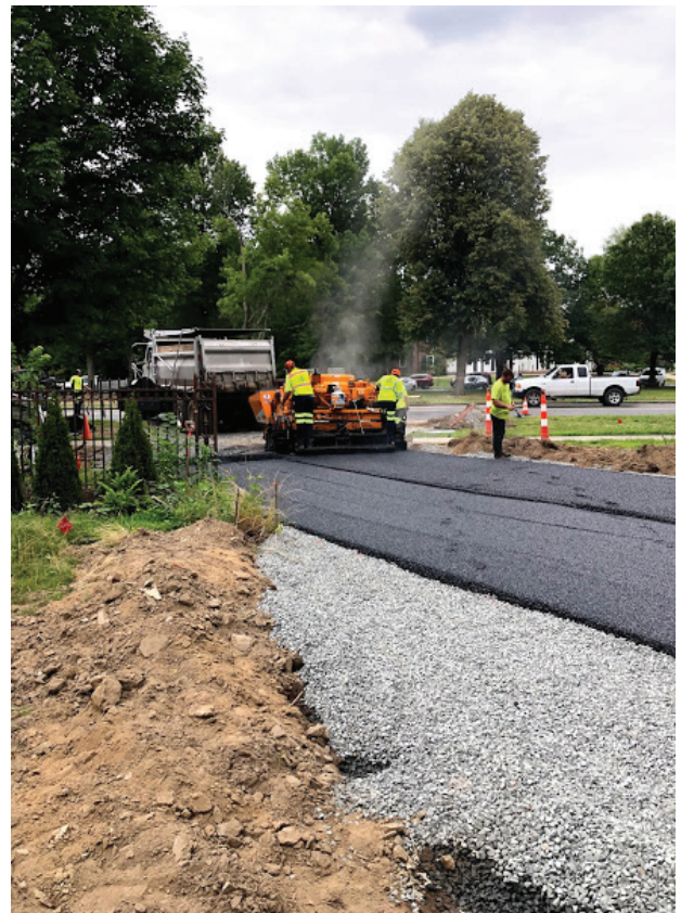
The driveway at the Brewer-Young Mansion paved with SmartMix reacted tire rubber
