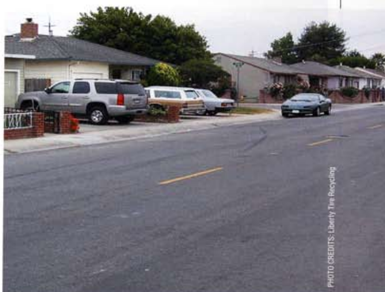
AR/PMAR three-layer cape seal after six years of performance, spring 2009, same location.
